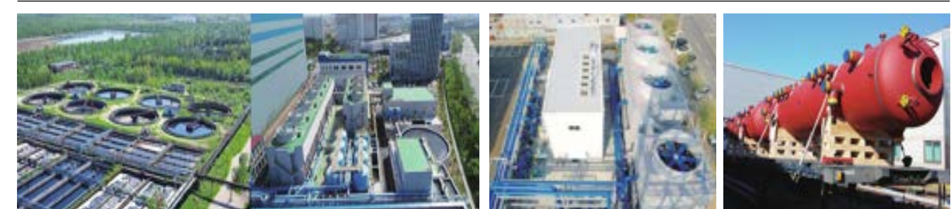
Water Treatment System
